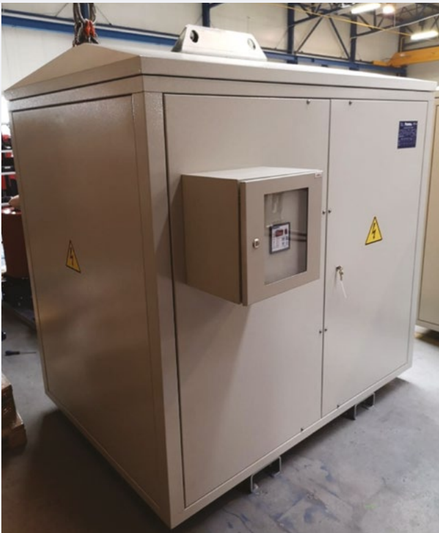
1600 kVA 11/0,705–0,403 kV 60 Hz IP 54 cast resin transformer installed on oil rig in Scotland
